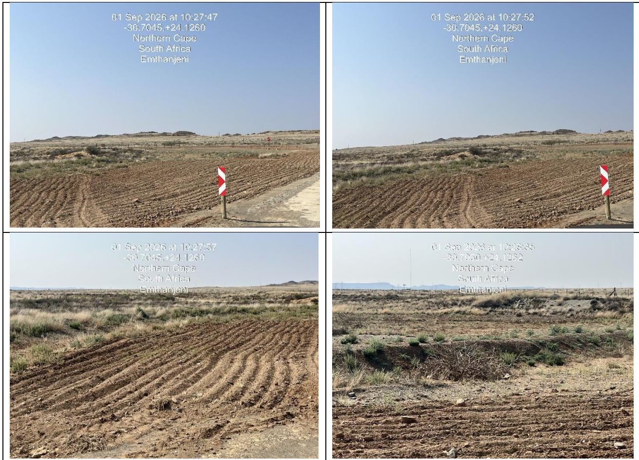
Photo Plate 2: Access Road
